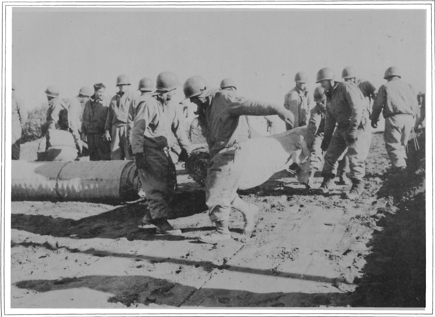
Men of the 540th Engineers lay matting for a temporary road on the beach near Nettuno.
